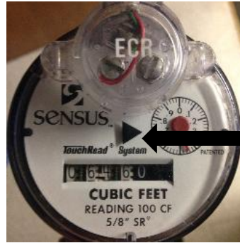
Leak Indicator: Black Triangle in center of the meter
